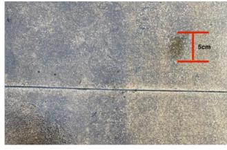
*Figure 18.* The photo of small ponding of 5 cm in length was taken on February 11<sup>th</sup>, 2024.
