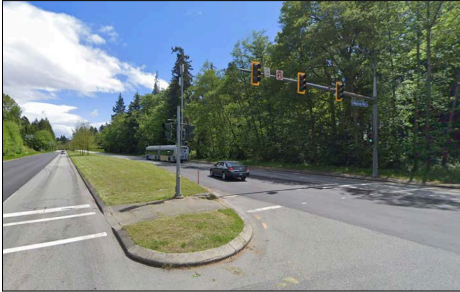
Figure 9. Crossing Signal Existing Example
