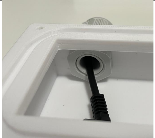
Figure 55: Put the locknut from the other side of the hole and tighten to secure the cable gland.
